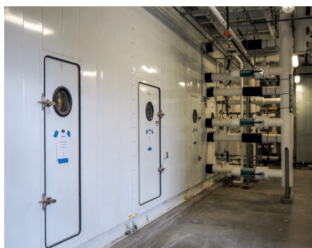
External view of the ventilation unit including the piping for the high performance closed circulation system from Konvekta.
