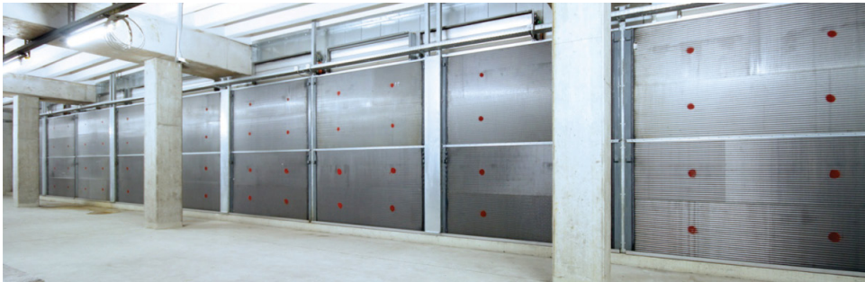
New heat transfer wall from Konvekta in the supply air station for basic heating of outside air to constant 60 °F. (Photo: Kulle & Hofstetter)
