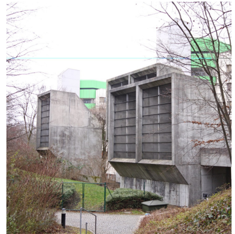
Central outside air intake to supply the hospital's HVAC system (Photo: Konvekta AG)
