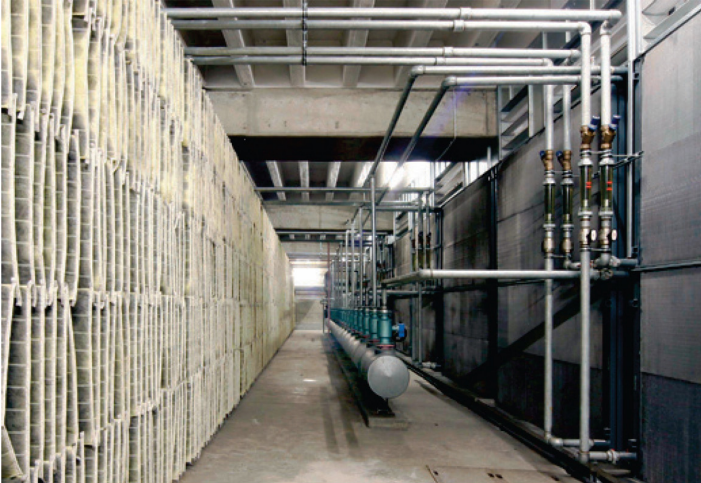
New heat transfer wall from Konvekta and air filters (Photo: Kulle & Hofstetter)
